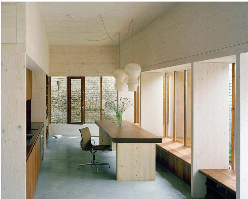
*'Off-site manufacture of the two timber packages comprising the majority of the building fabric resulted in reduced waste, better cost control and excellent quality of finish whilst the frame embodies 17 tonnes of stored CO<sub>2</sub>'*
