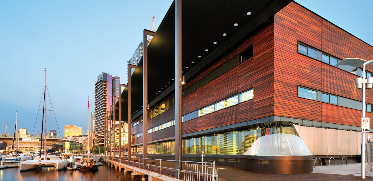
Library at the Dock, Melbourne - helping tackle climate change by storing 250 tonnes of carbon in its wood
