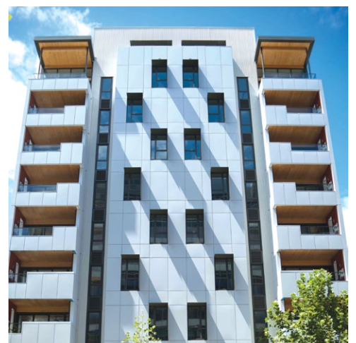
Forte, Melbourne - 10 storeys of cross laminated timber, built in 3 months with just 4 workers and a crane driver.
